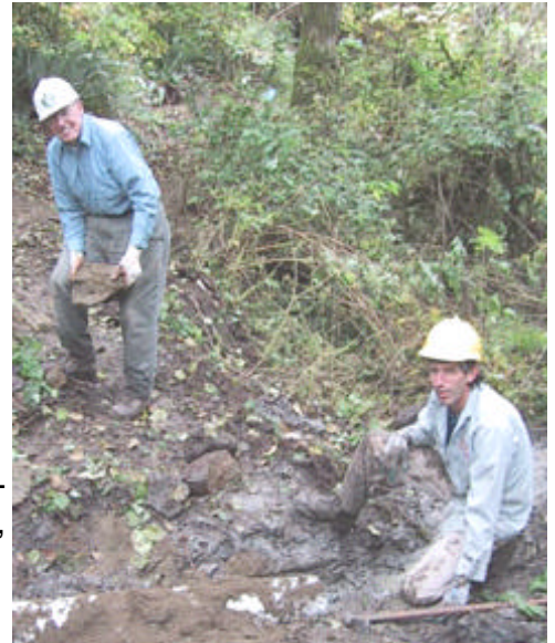
Trail veterans Duane Acheson and Jim Oosterhof construct rock headwall for culvert installation near
